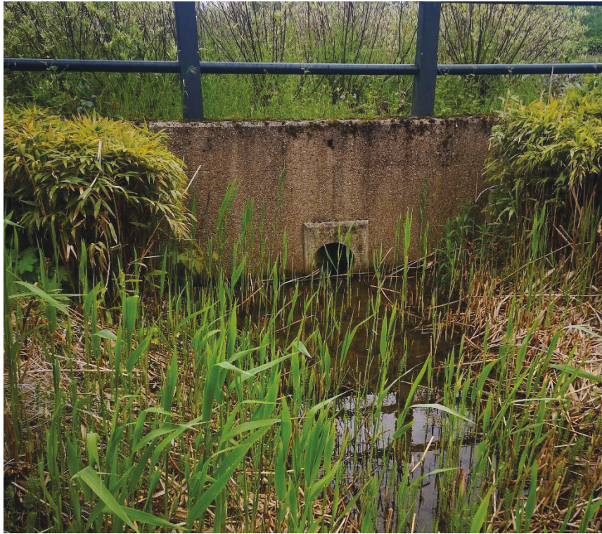
Figure 4.23: The swale outlet pipe at Upton. (Copeland-Phillips, 2021)
