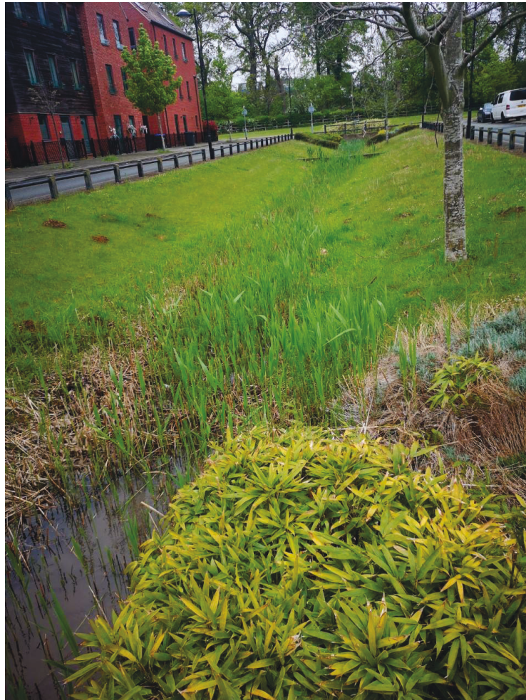
Figure 2.5: Example of a vegetated swale, Upton, Northampton (Copeland-Phillips, 2021).
