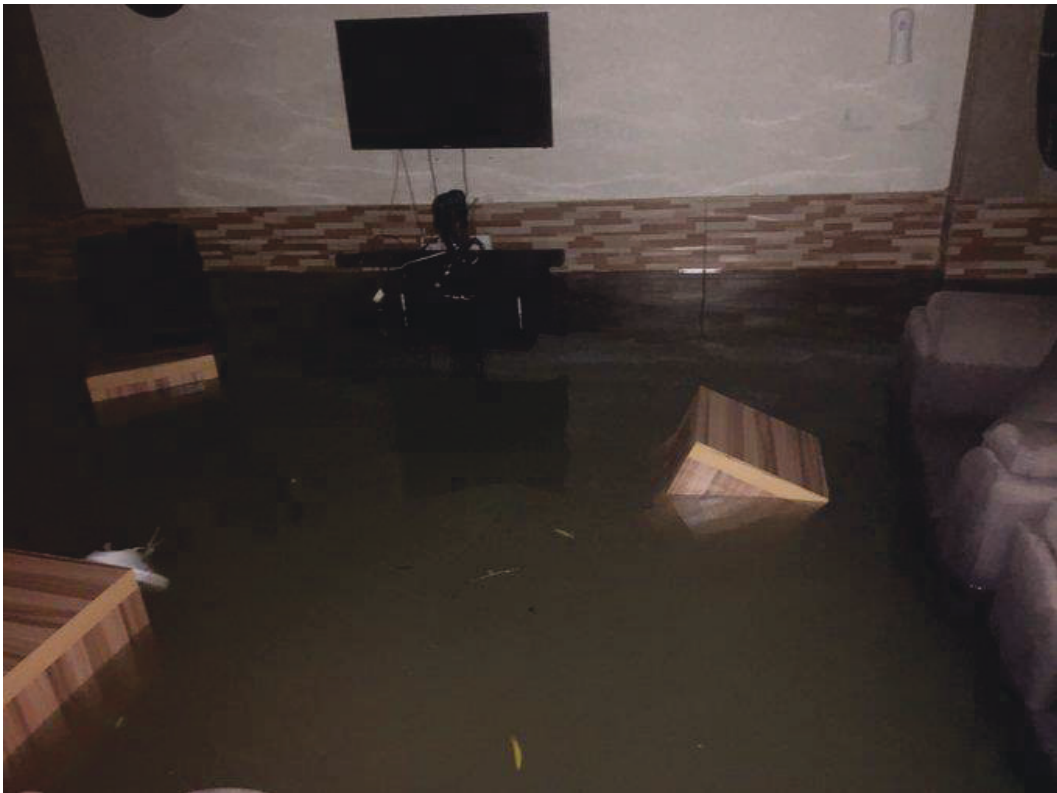
Figure 3.15: Flood waters inside Residential Property in Lekki, Lagos
