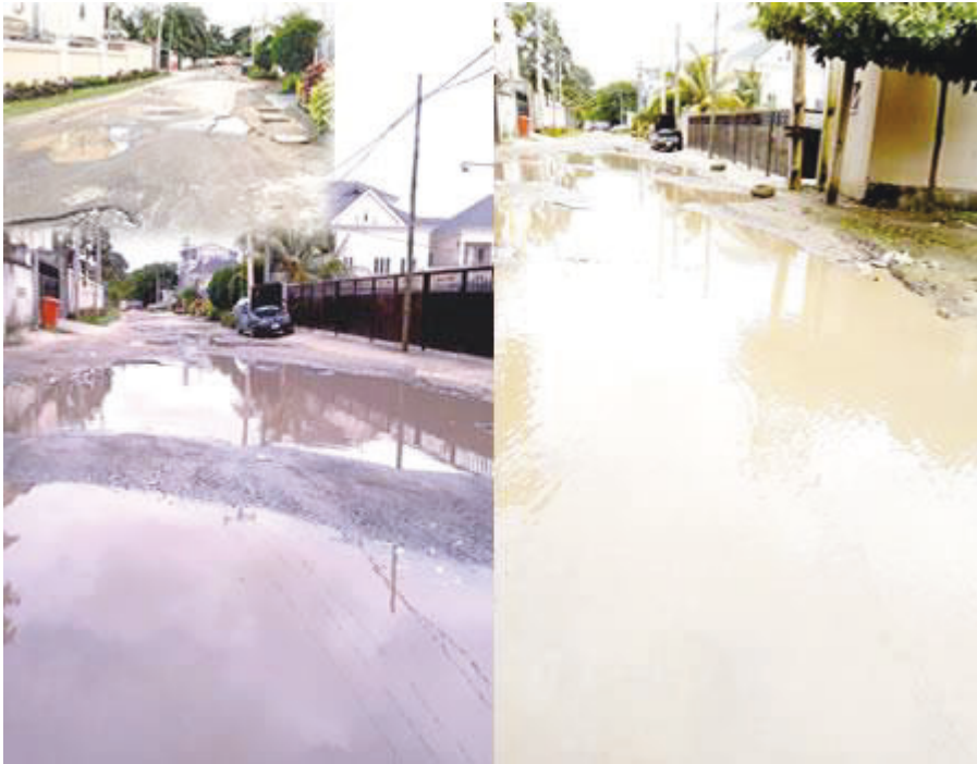
Figure 3.3: Flooding in Ikeja GRA, Lagos
